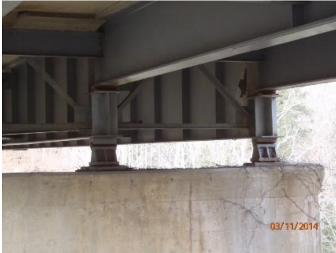
View of the north bearings over pier 4.
