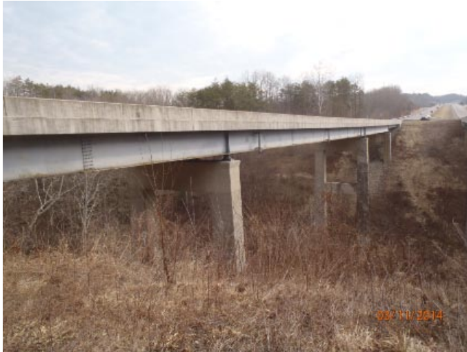
View from the south near abutment 1.
